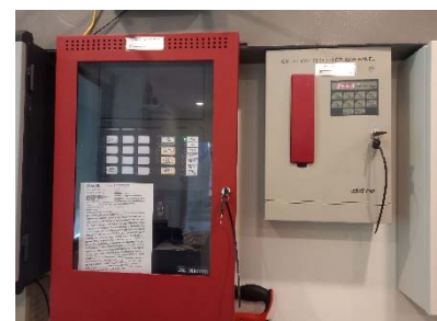
Fire Fighter Telephone System
